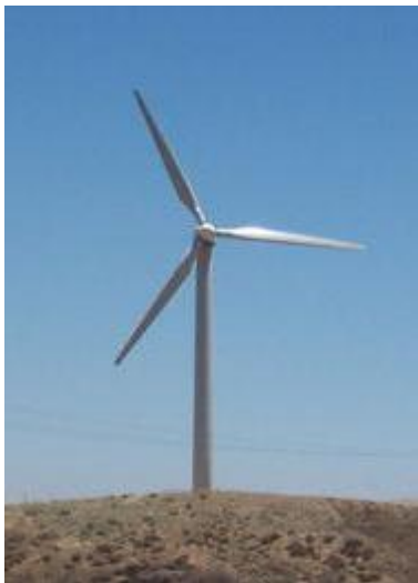
Figure 1: The horizontal-axis wind power turbine.
